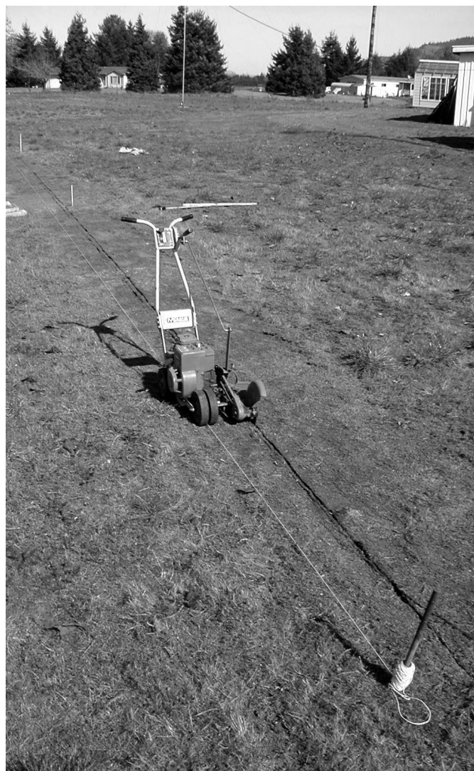
Figure 19 — Cutting a slot in the soil for the 40 foot buried dipole.
