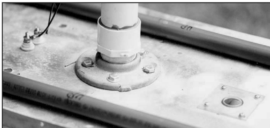
Figure 3—Galvanized pipe floor flanges are used top and bottom to connect the mast and crossover feed support. This is the top flange with a PVC adapter. The hole to the right of the flange is for a coaxial feed line for the 2-meter quad mounted above the W8JK array. Ceramic feedthrough insulators on left are for the 450 Ω ladder line feed.
