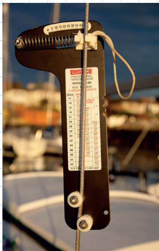
This Loos gauge is indicating that the 6mm wire in the cap shroud is at 22% of its breaking strain (730kg)
